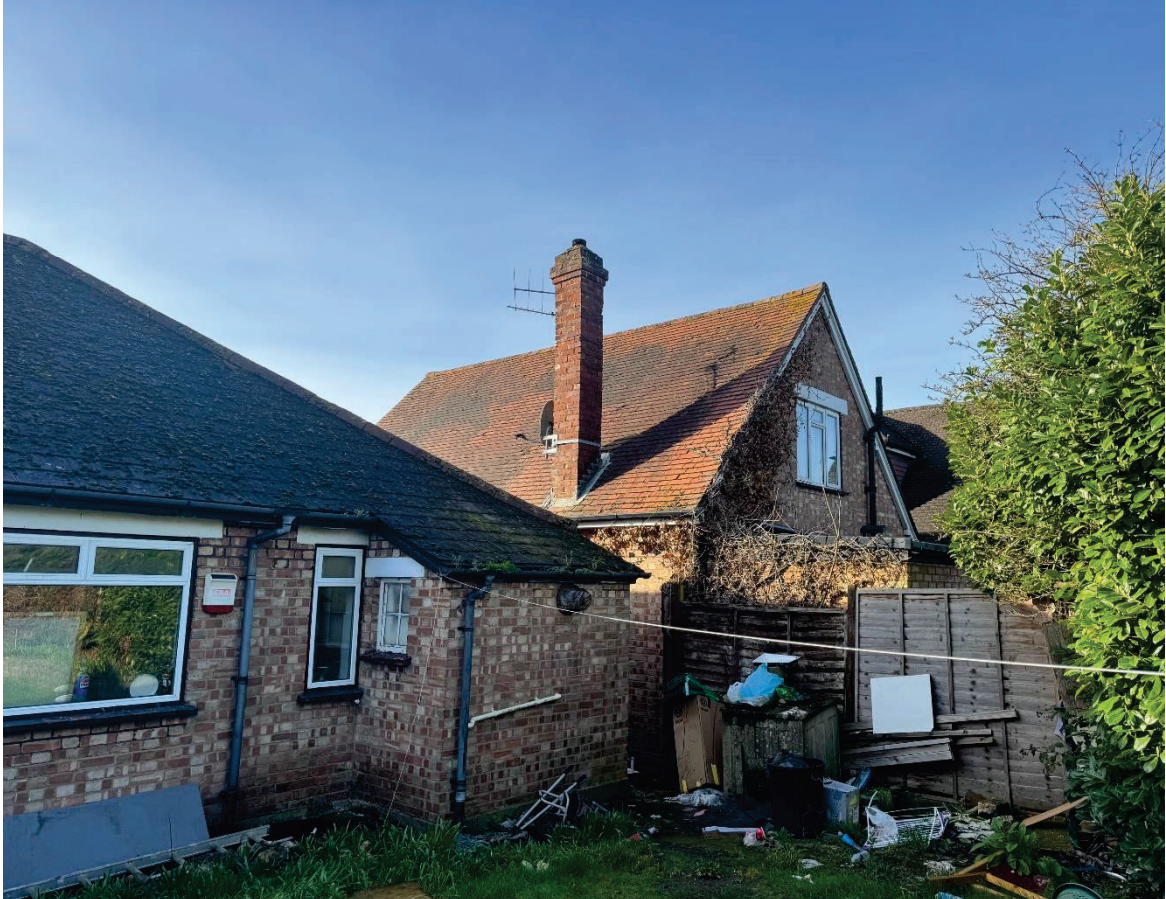
Figure 5 – Rear view of No.27 Clammas Way from application site
