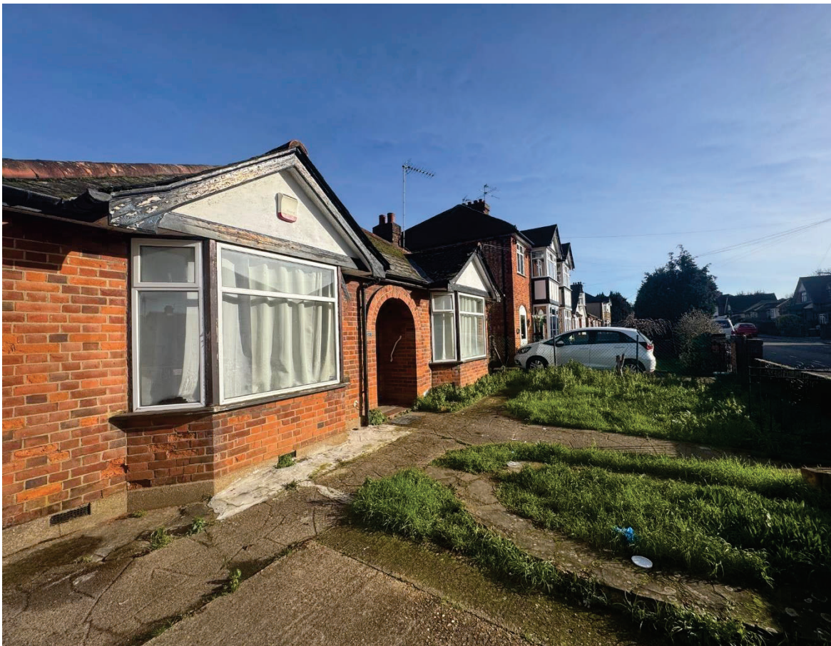
Figure 7 – Existing Site Frontage
